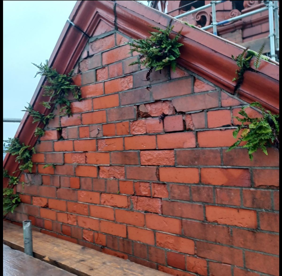
Gable End wall
