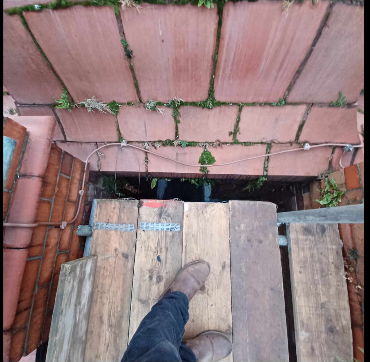
Small arch / chimney / gable wall
