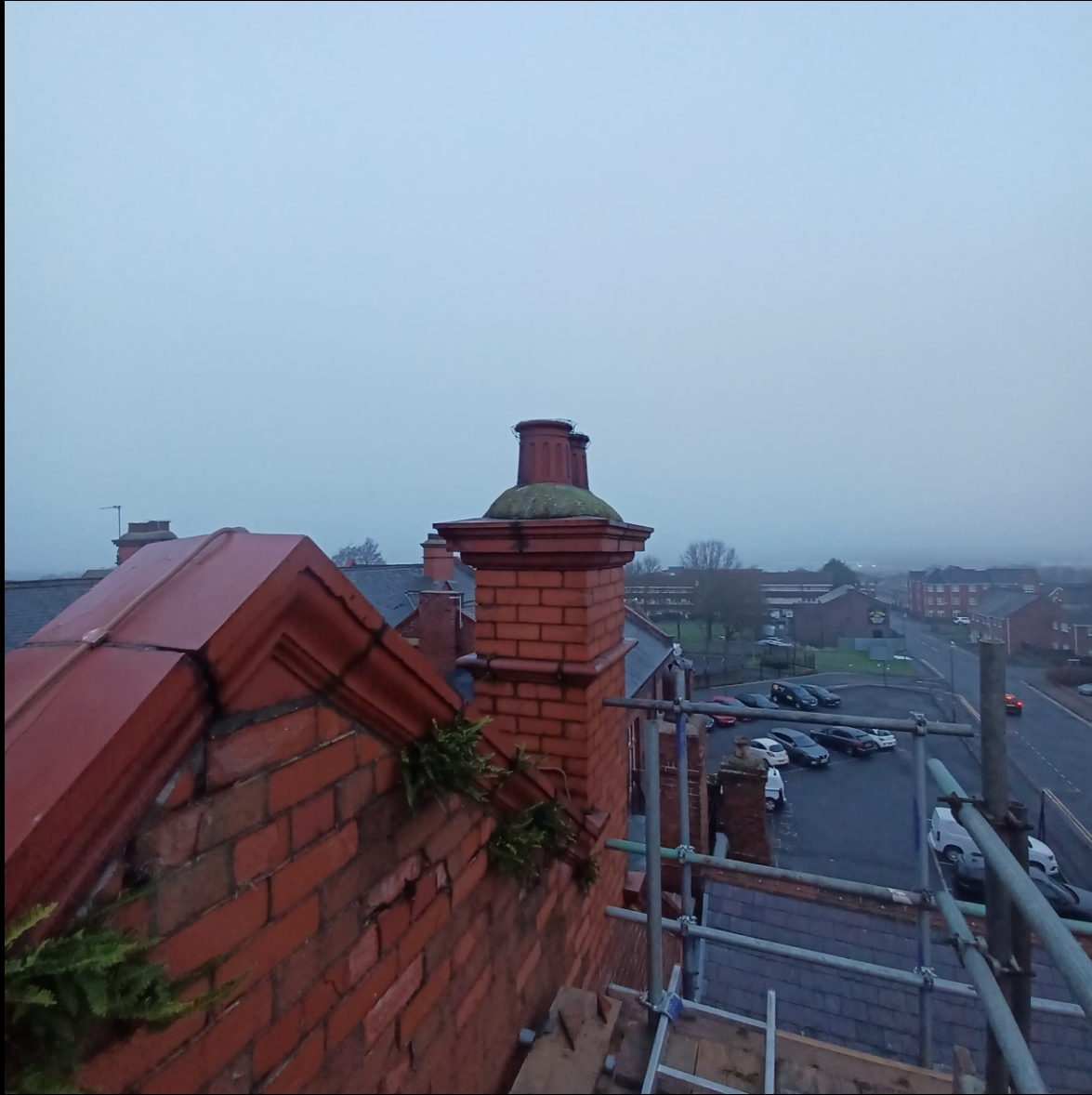
Gable wall facing to rear, showing 2 nd chimney stack
