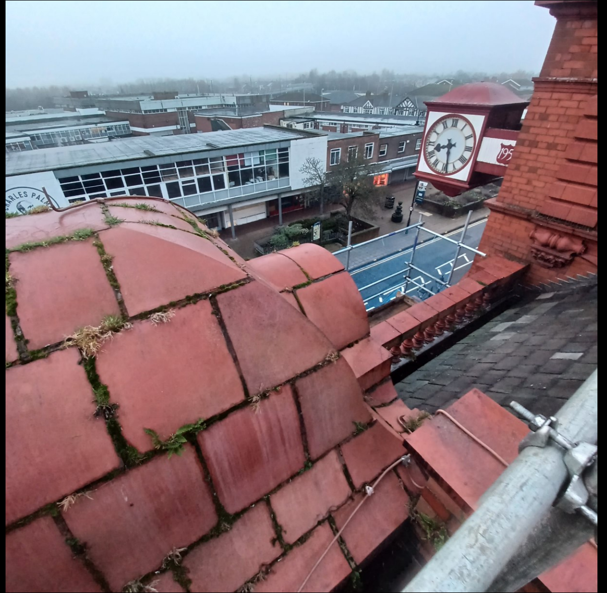
View from above small arch and parapet wall
